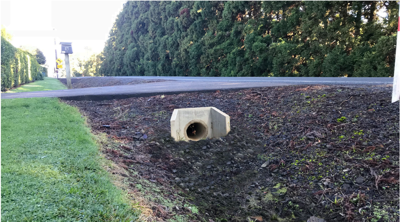
Dangerous concrete headwall – potential fatality to errant vehicle
