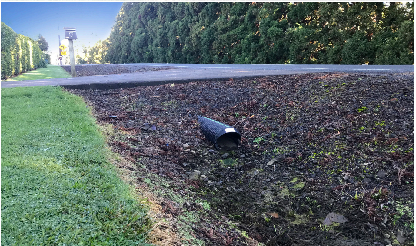
CyclopsShield™ Replacement – Safe traversable end for errant vehicle
