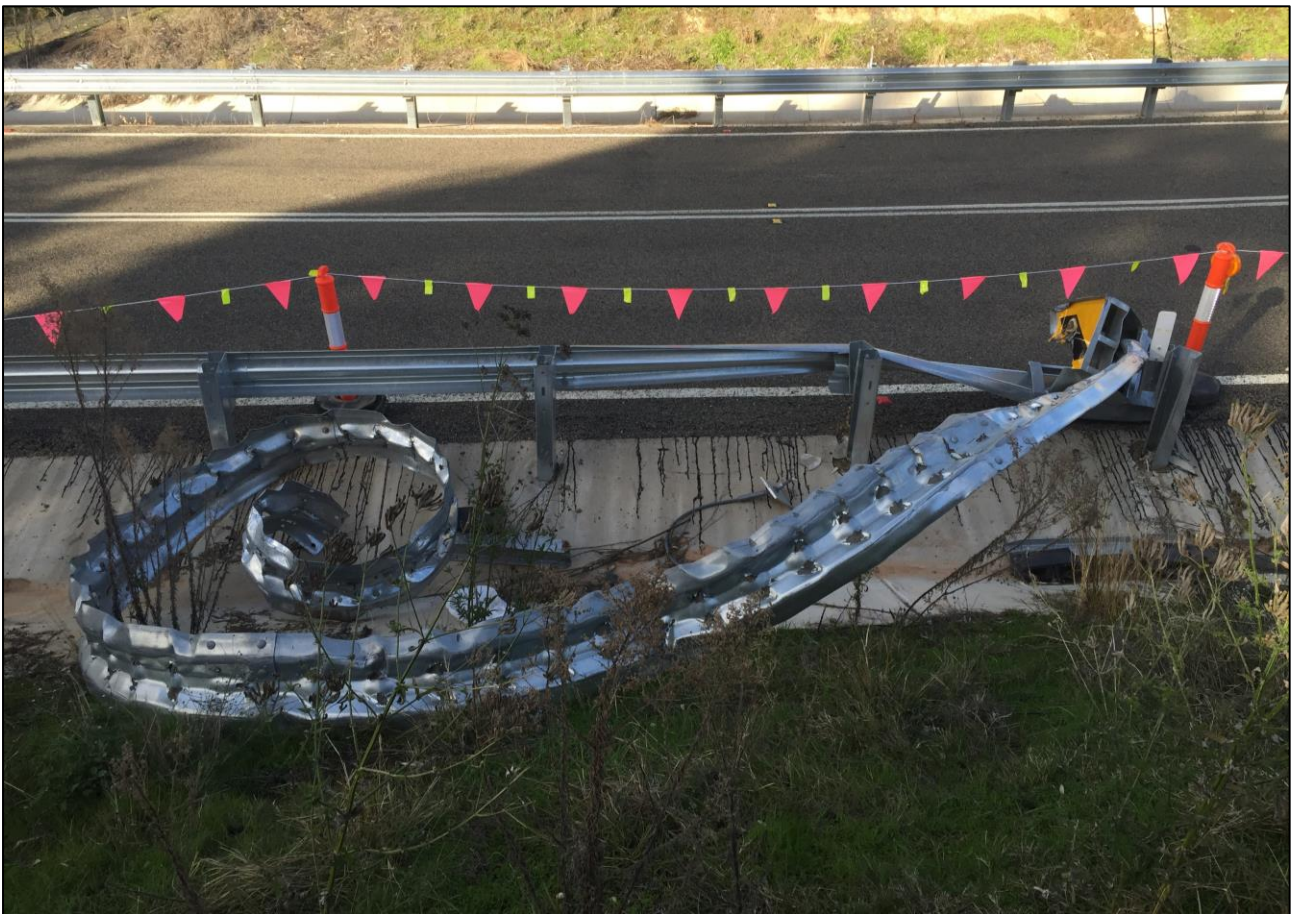
Damaged Rail after Travelling through Impact Head
