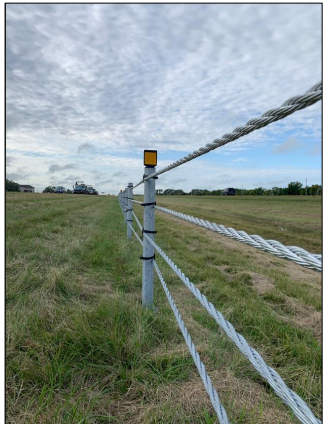
Figure 14: Line Post Assembly
