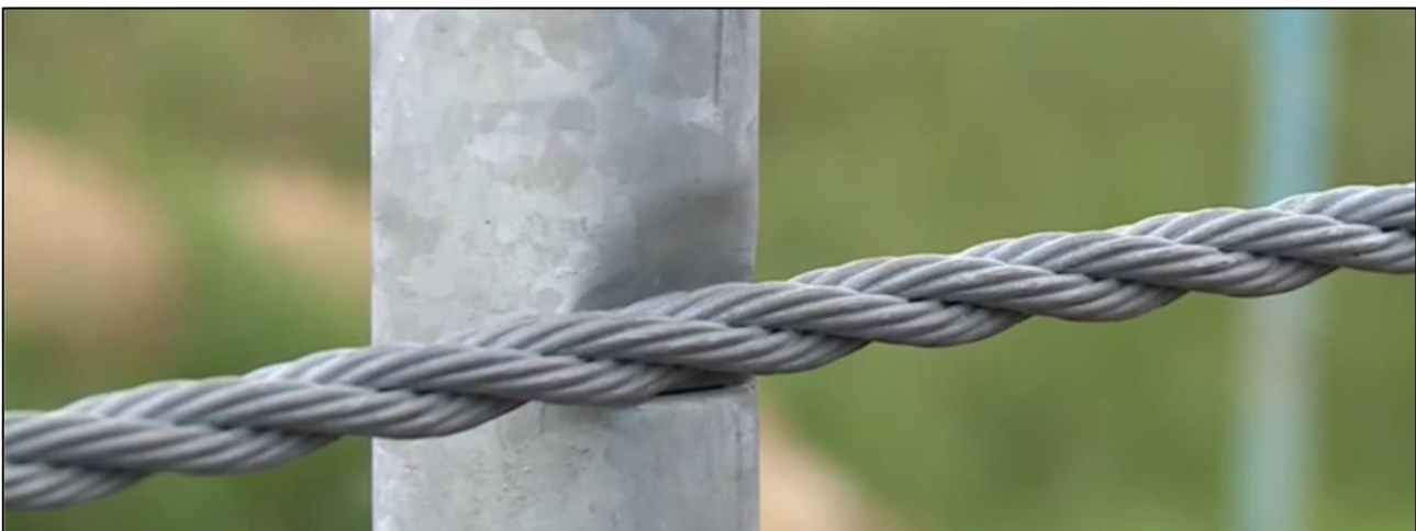
Figure 7: Rope Located within Recess of Line Post before Attachment of Retainer Clip
