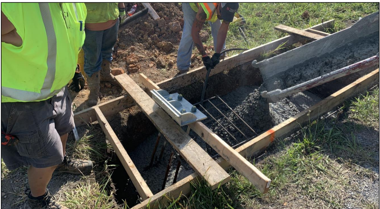
Figure 1: Placement of Anchor Plate
