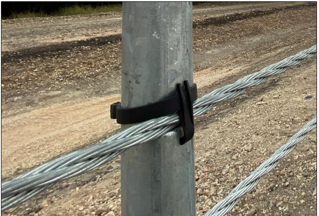
Figure 10: Retainer Clip Position
