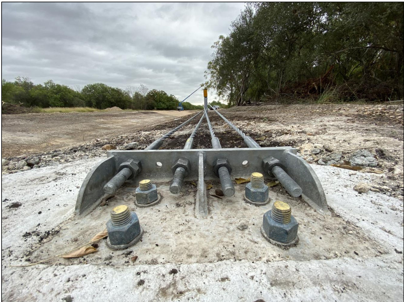
Figure 12: Anchor Bracket Assembly
