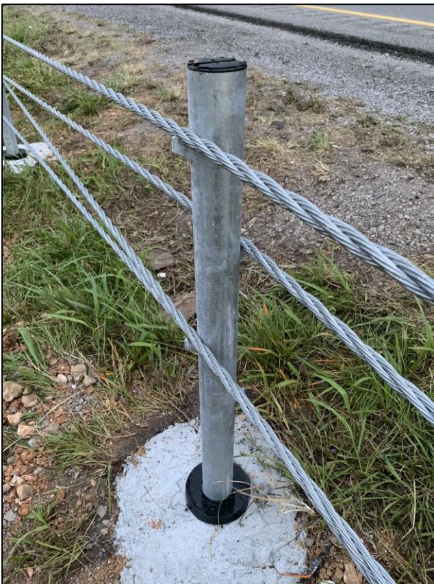
Figure 14: Deflection Post Assembly
