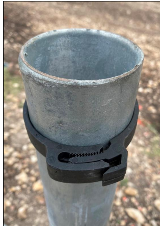
Figure 9: Securing of Retainer Clip
