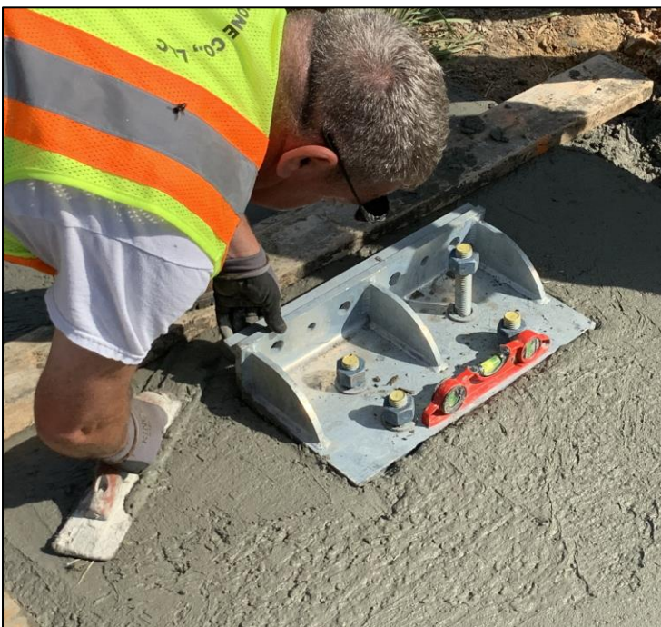
Figure 3: Levelling Anchor Plate
