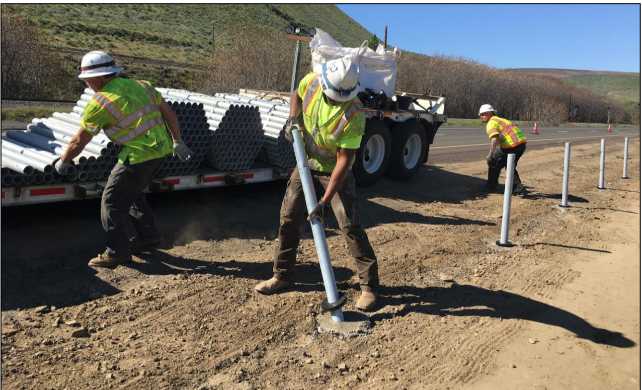
Figure 6: Installation of Line Posts
