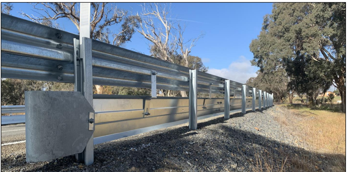
Figure 5: Attachment of Bullnose (rear views)
