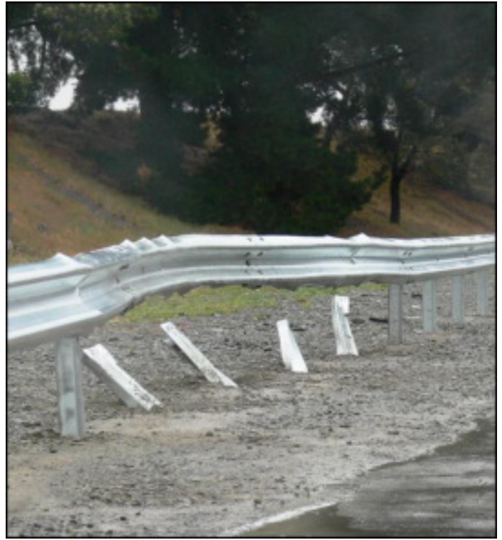
Figure 3: Controlled release of rail during impact
