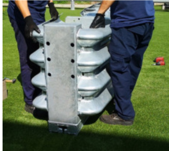
Fig. 20: Positioning of the new trolley
