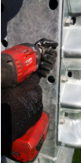
Fig. 18: Unscrewing of the trolley
