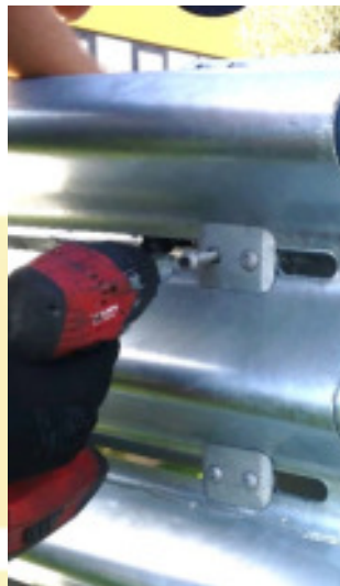
Fig. 16: Removal of the sliding element
