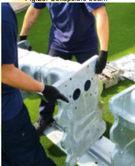
Fig. 26: Replacement of the collapsible beam
