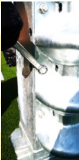
Fig.15: Removal of the threaded bar
