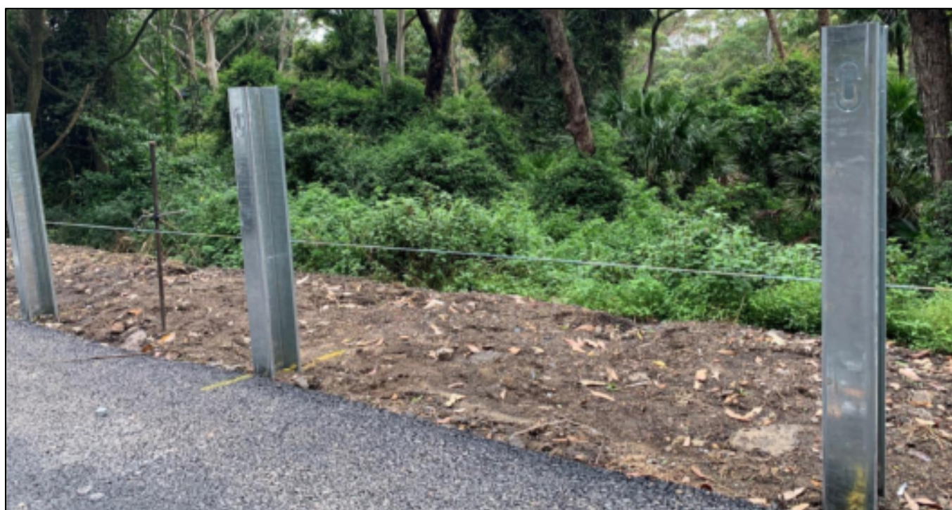
Figure 6: RamShield® HC Post Installation
