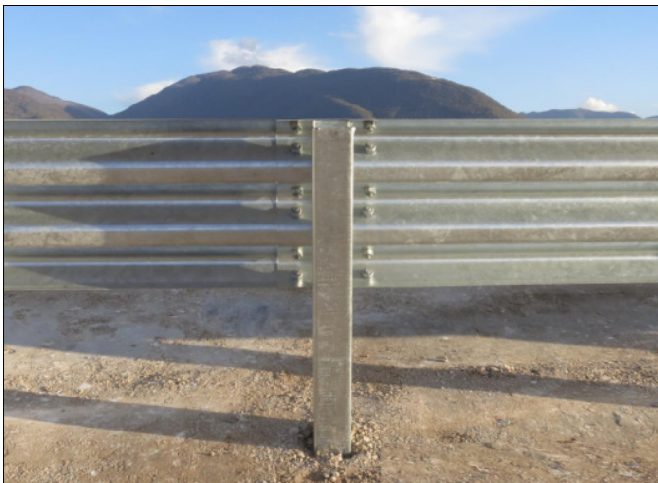
Figure 7: Splice Arrangement
