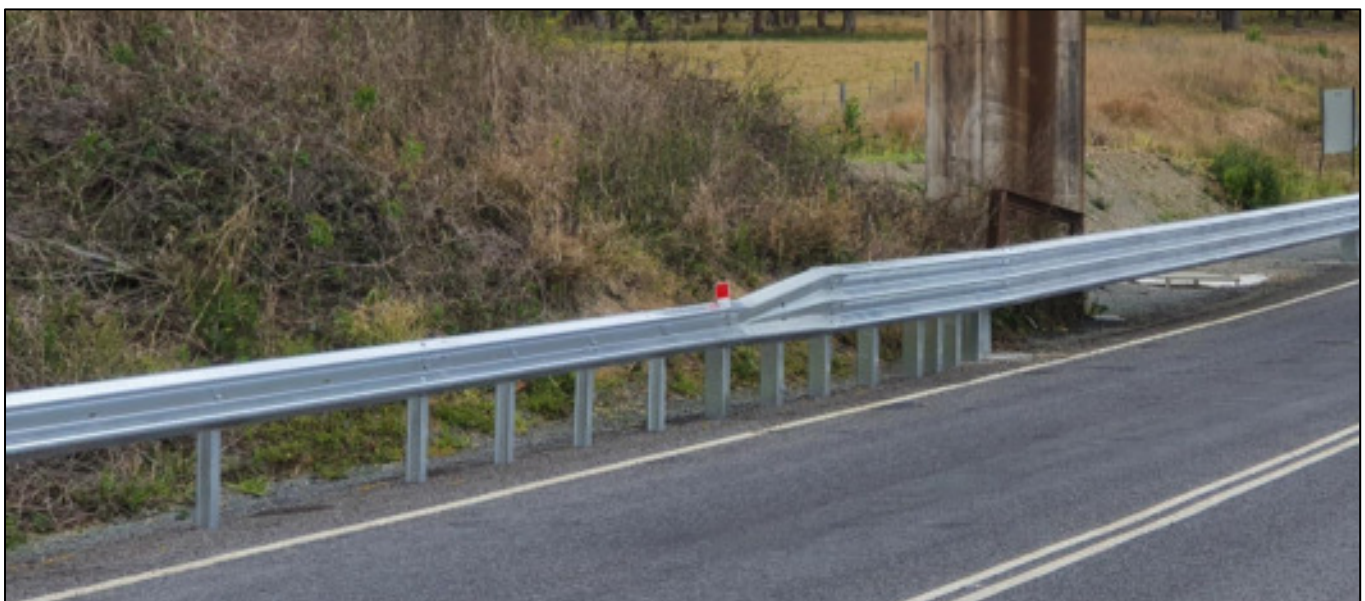
Figure 5: CrocGuard® Connection to RamShield® W-Beam
