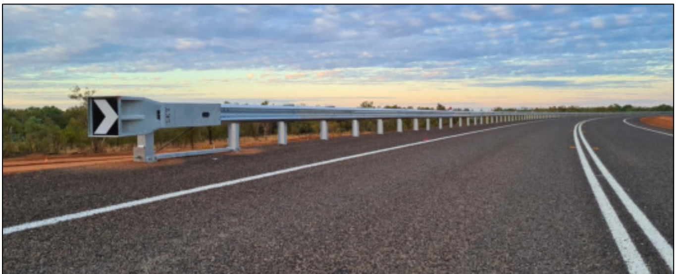
Figure 7: CrocGuard® Connection to MSKT Terminal
