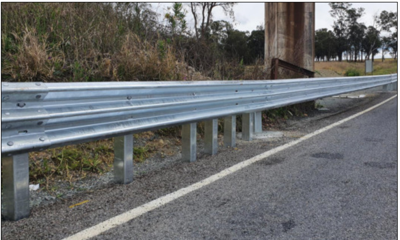
Figure 6: CrocGuard® Connection to RamShield® HC
