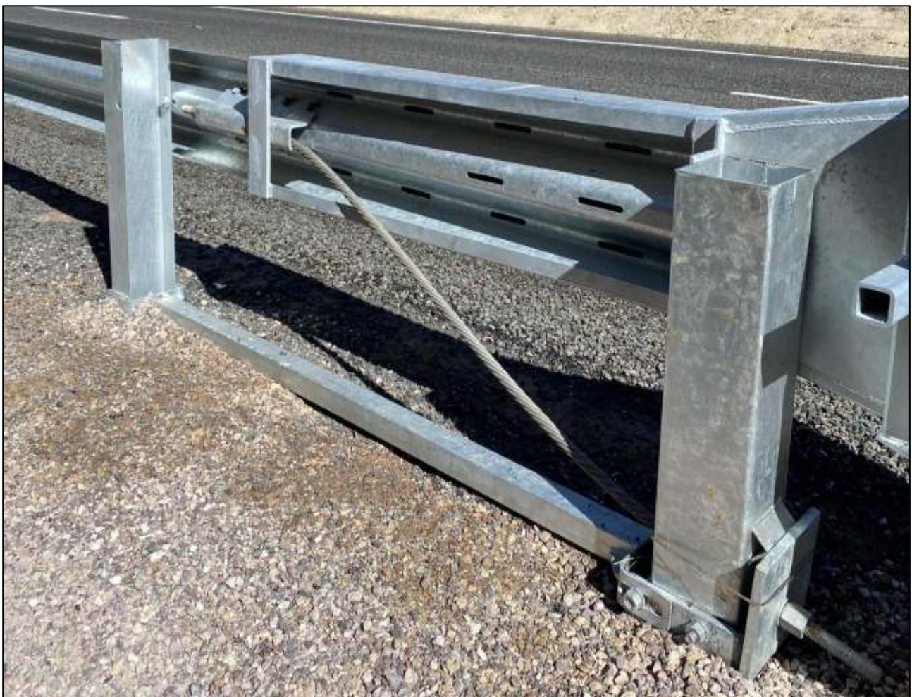
Figure 12: MSKT Anchor Assembly – Rear View
