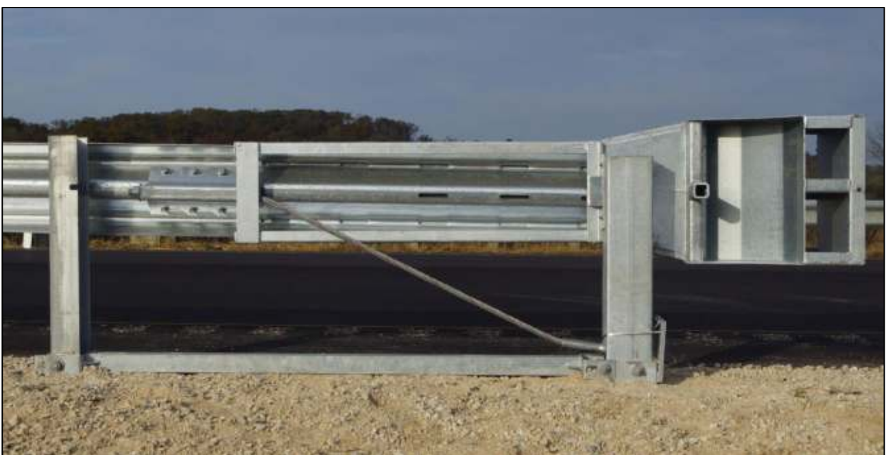
Figure 9: Attachment of Cable Anchor Bracket
