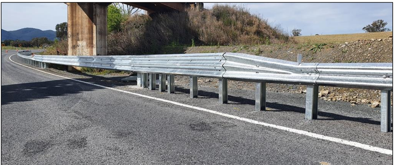
Figure 10: Connection to CrocGuard® (Departure View)
