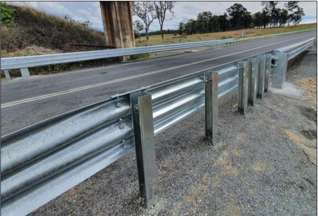
Figure 12: Thrie-Beam Connection to Transition Posts
