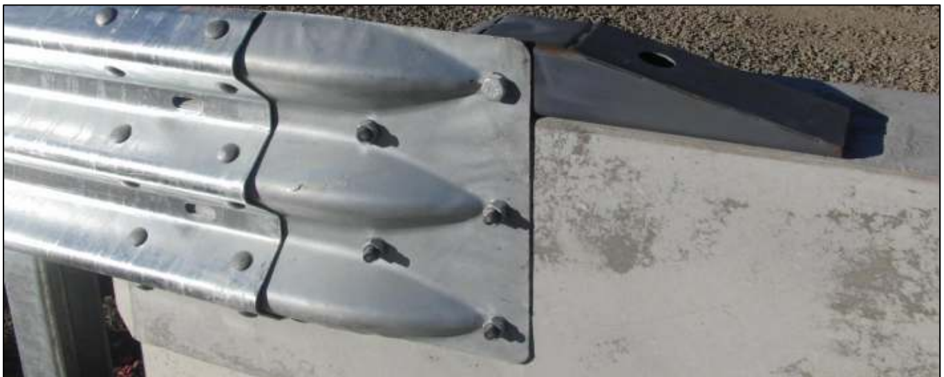
Figure 11: Thrie-Beam Terminal Connection to Top Mount Bracket
