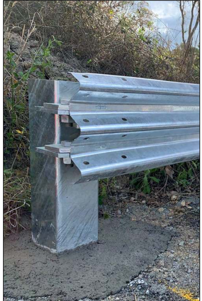
Figure 9: CrocGuard® Abutment Post
