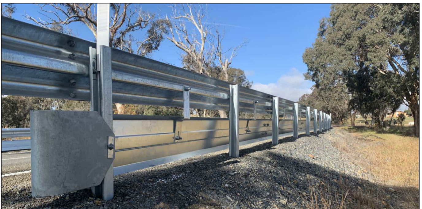
Figure 5: Attachment of Bullnose (rear views)
