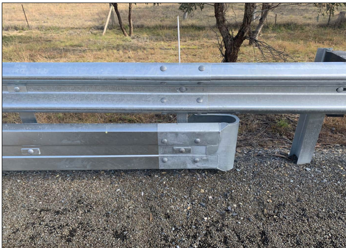
Figure 4: Termination of BikerShield™ in advance of Guardrail End Terminal Posts
