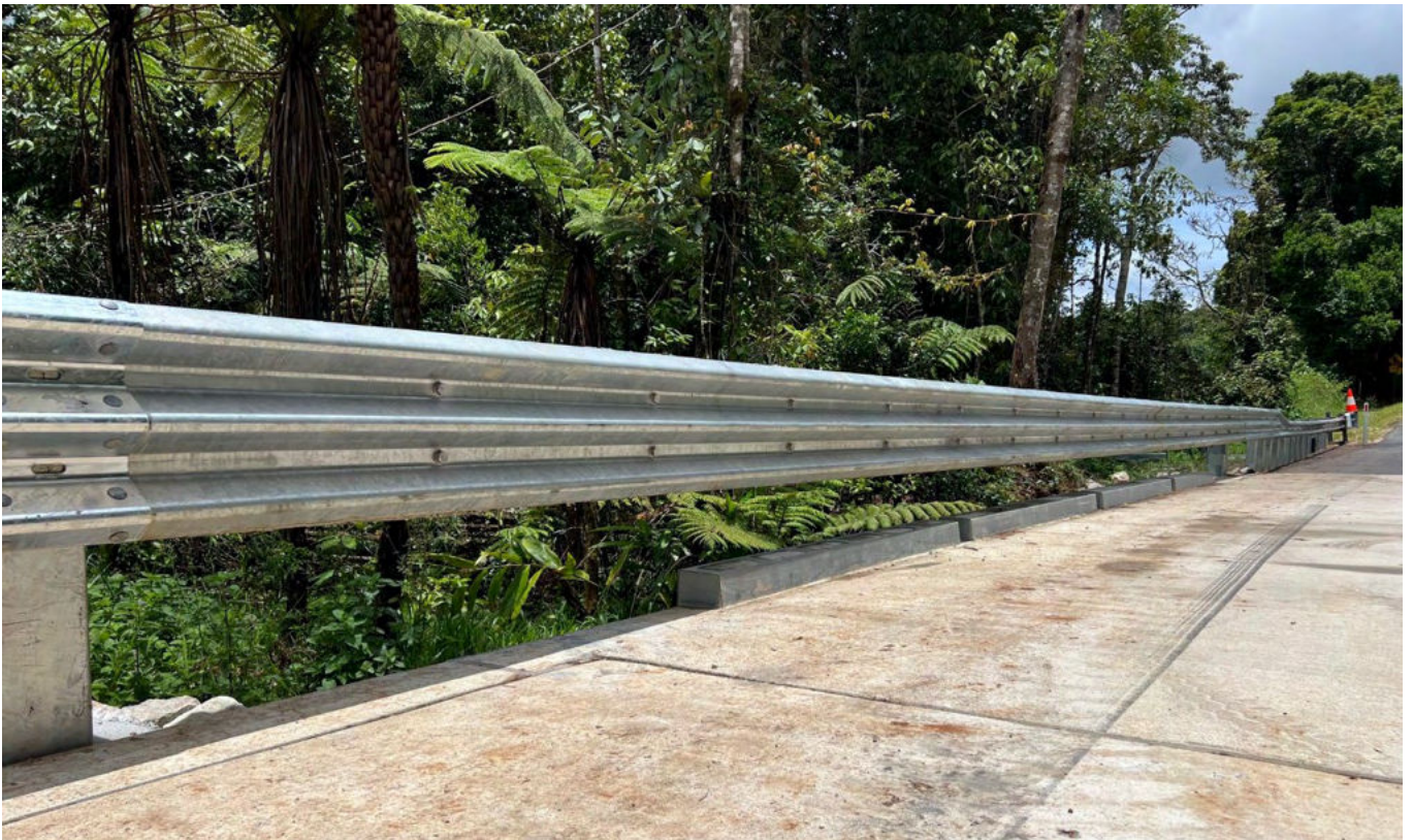
Figure 6: CrocGuard® Connection to RamShield® HC
