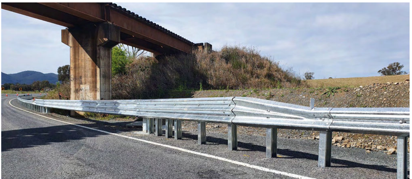
Figure 5: CrocGuard® Connection to RamShield® W-Beam
