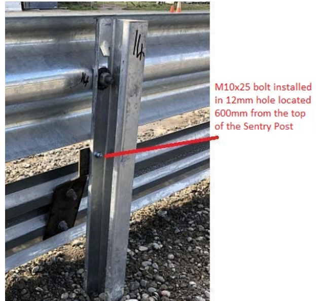
Figure 2. ACP Sentry Barrier: Attachment of Mounting Bracket.
