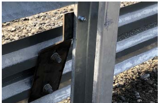
Figure 3. ACP Sentry Barrier: Mounting Bracket attached (rear view).
