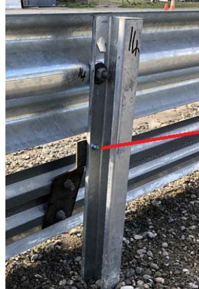
Figure 1. ACP Sentry Barrier: Attachment of Mounting Bracket.
