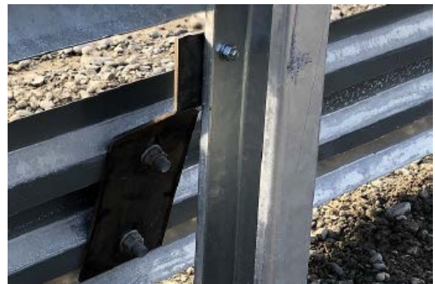
Figure 2. ACP Sentry Barrier: Mounting Bracket attached (rear view).
