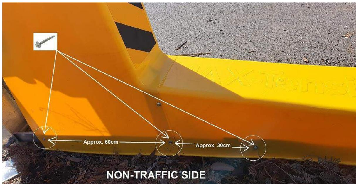
15.6 Re-tighten the frontal cable assembly nuts to secure the plastic to the ground strut. Ensure the washers are on the outside of the plastic.
