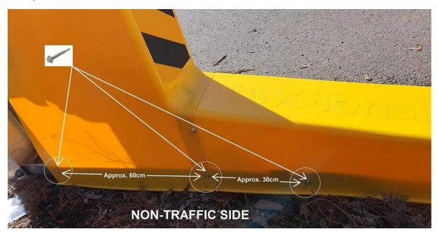
15.6 Re-tighten the frontal cable assembly nuts to secure the plastic to the ground strut. Ensure the washers are on the outside of the plastic.
