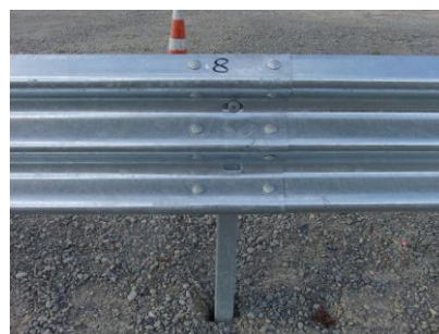
Splice Joint location
