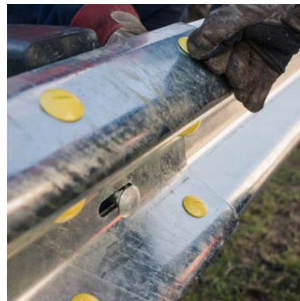
Figure 12. Splice rail 2 to rail 3 with 8 special shear bolts
