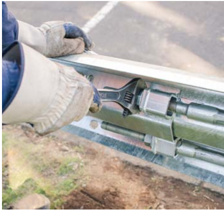
Figure 28. Tighten cables at Cable Bracket end (post 7)
