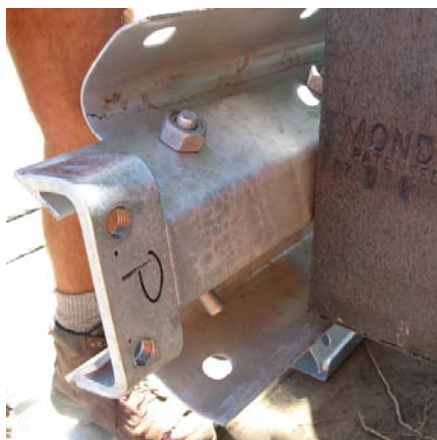
Figure 13. Bolt Slider Bracket to end of rail 2 at post 3
