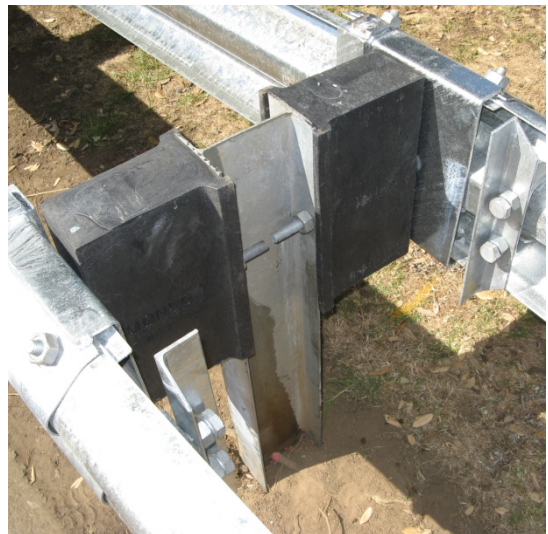
Figure 36. Re-attach the angle bar to the Slider Bracket
