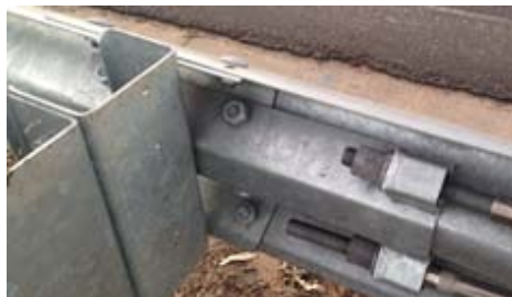
Figure 10. Cable Anchor Bracket on back of rail 3
