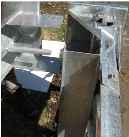
Figure 30. Fit secondary head to main head
