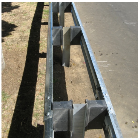
Figure 32. Rails installed with blockouts
