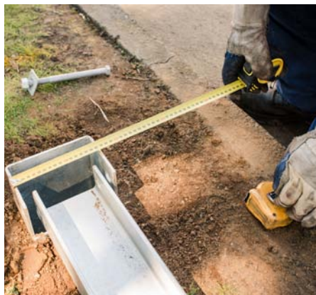
Figure 7. Measure 200mm towards roadway
