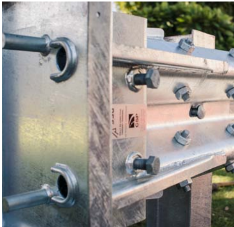
Figure 20. Attach Impact Head to rail 1
