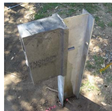
Figure 6. Bolt the blockout prior to attaching the rail
