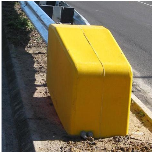
Figure 38. Attach nose cone using cable nuts
