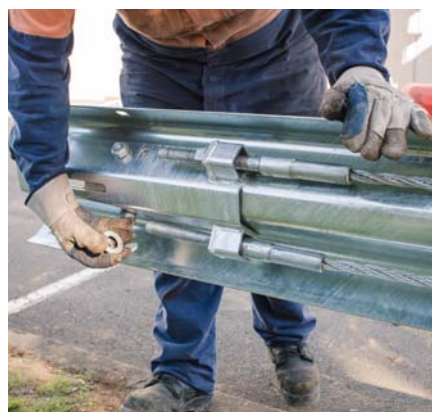
Figure 25. Do not tighten nuts at this time
