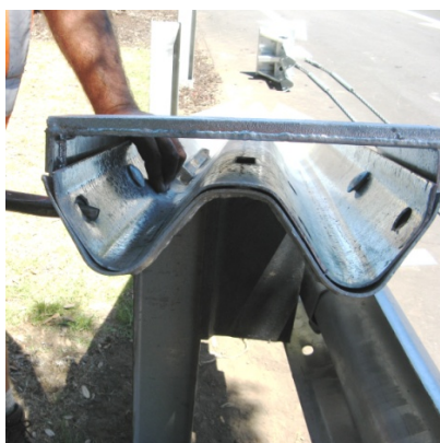
Figure 15. Sit rail 1 so it is raised off the ground
