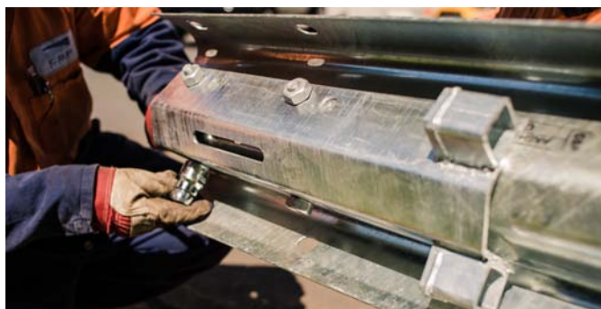
Figure 10. Cable Anchor Bracket on back of rail 3
