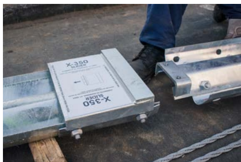
Figure 17. Push Slider Panel over rail 2
