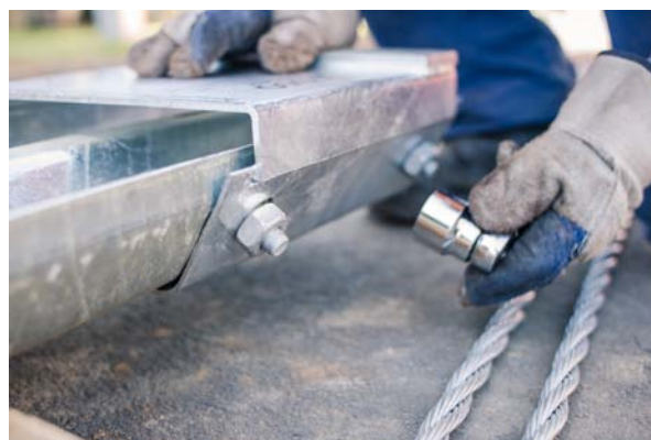
Figure 16. Slide the Slider Panel onto downstream end
