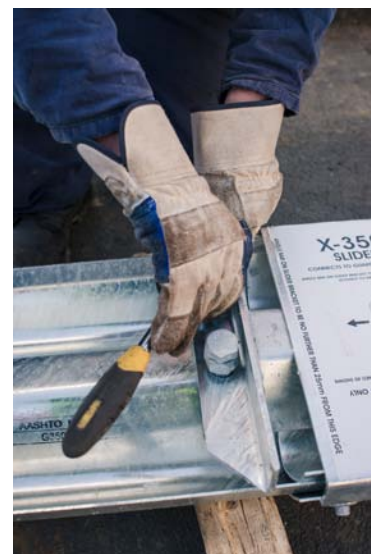
Figure 19. Reattach the angle bar
