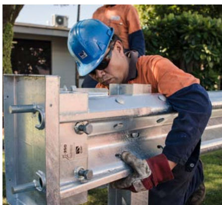
Figure 24 Pass the cable through the bottom hole
