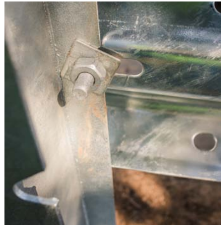
Figure 21. Bolt head and rail 1 to post 1 with washer
