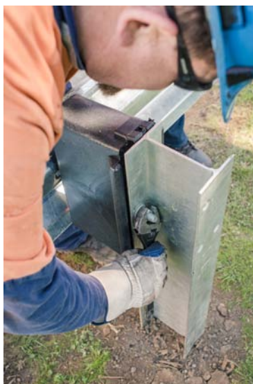
Figure 18. Bolt rail 1 and blockout to post 2
