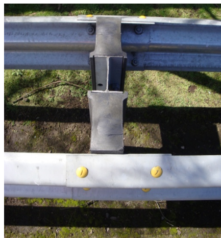
Figure 33. Splice rail 2 to rail 3 with 8 special shear bolts
