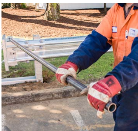
Figure 26. Use crow bar to turn Friction Plate
