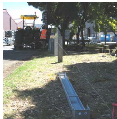
Figure 4. Pull a string line with the desired offset
