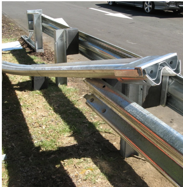
Figure 34. Fit the Slider Panel onto the straight end of rail
