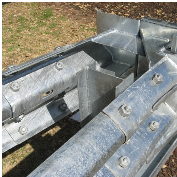
Figure 37. Use 8 standard splice bolts
