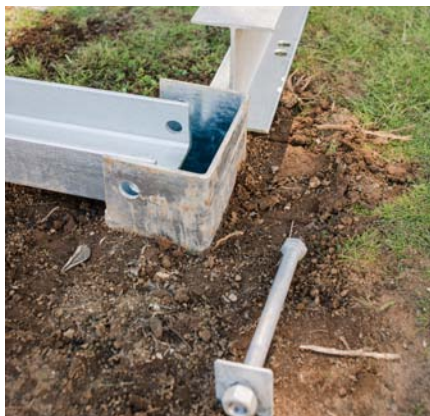
Figure 8. Drive soil anchor into augured hole
