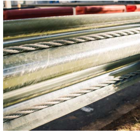
Figure 29. Tighten cables until they are taut
