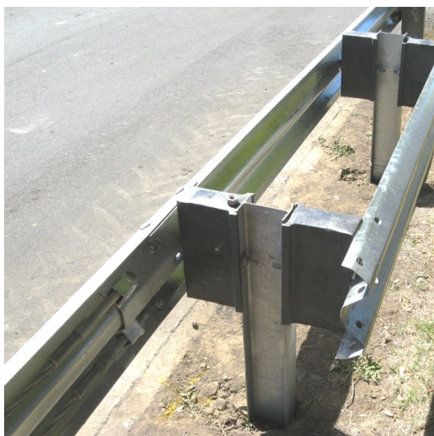
Figure 2. Essentially a tangent system installed parallel to Median barrier
