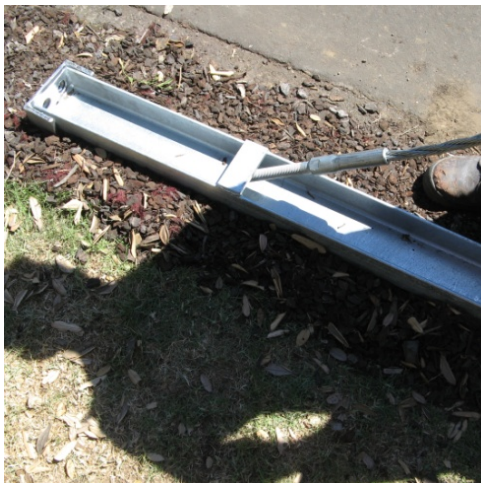
Figure 22. Push cables under steel strap on Ground Strut
