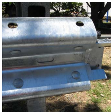
Figure 14. Remove angle bar bolts
