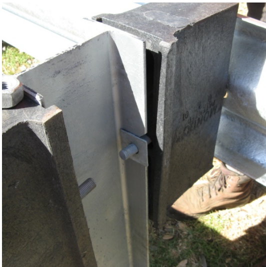
Figure 35. Bolt rail 1 and blockout to post 2 using the square washer
