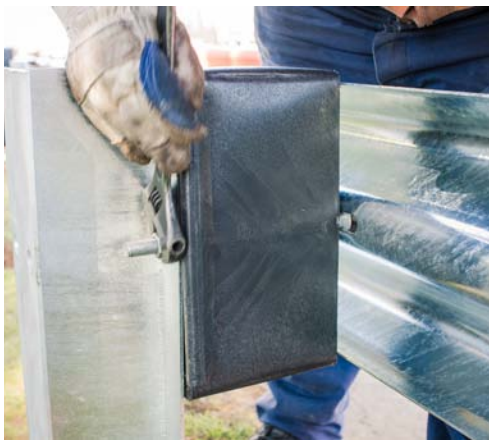
Figure 11. Bolt rail 2 to post and blockout
