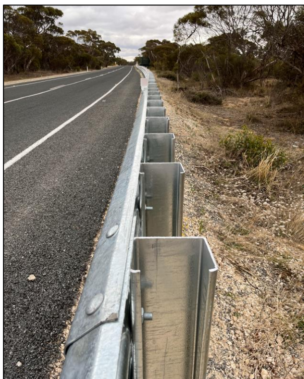
Figure 3: RamShield® HC Post Embedment Depth
