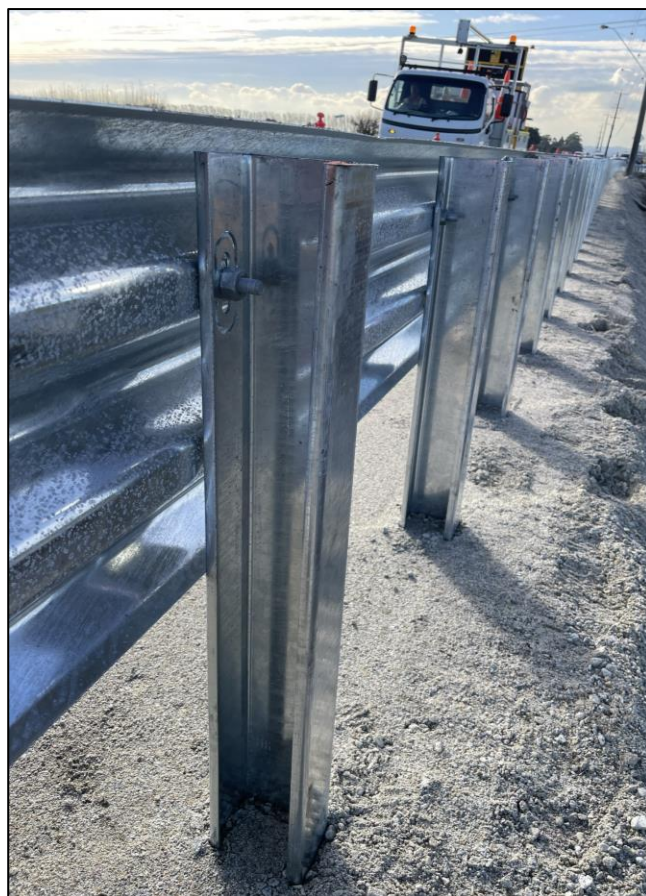
Figure 15: Post to Rail and Splice Arrangement
