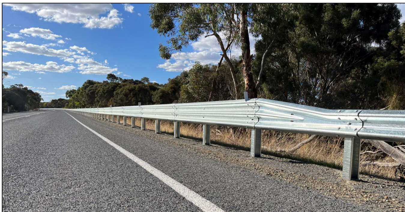
Figure 7: Installation of the Asymmetric Transition
