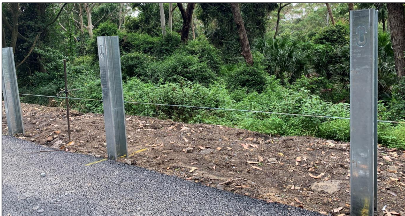
Figure 14: RamShield® HC Post Installation
