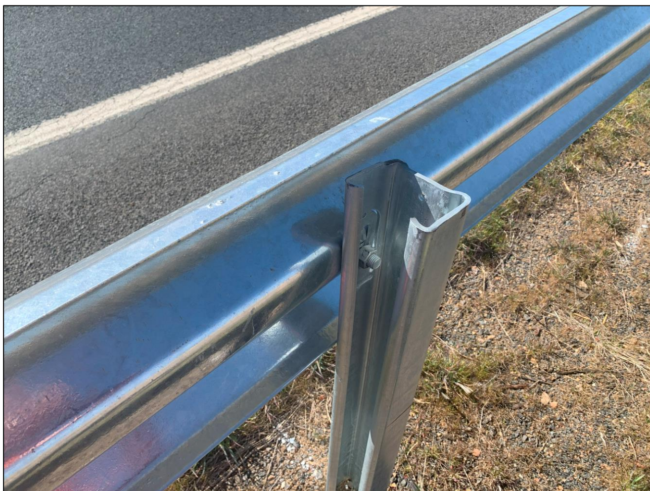
Figure 13: Attachment of W-Beam.
