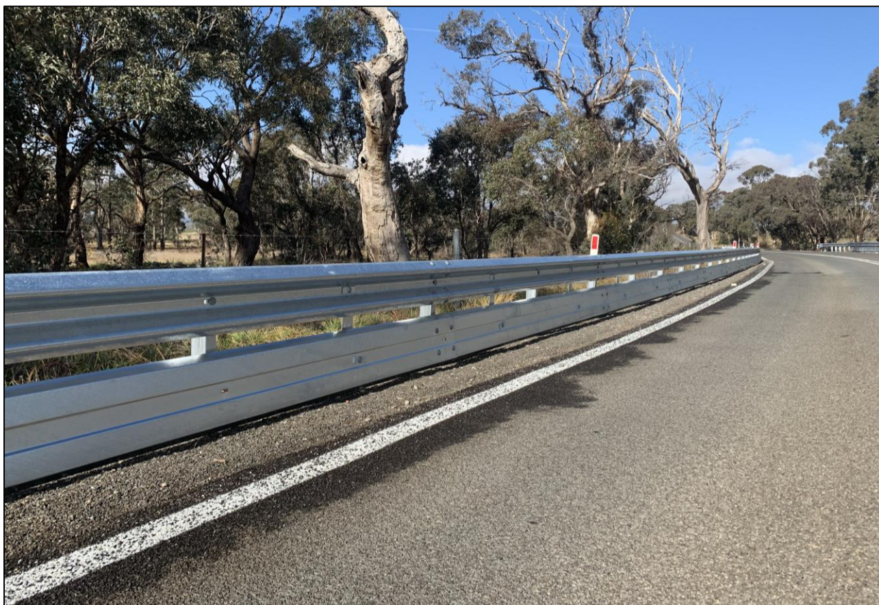
Figure 9: RamShield® W-Beam with BikerShield™
