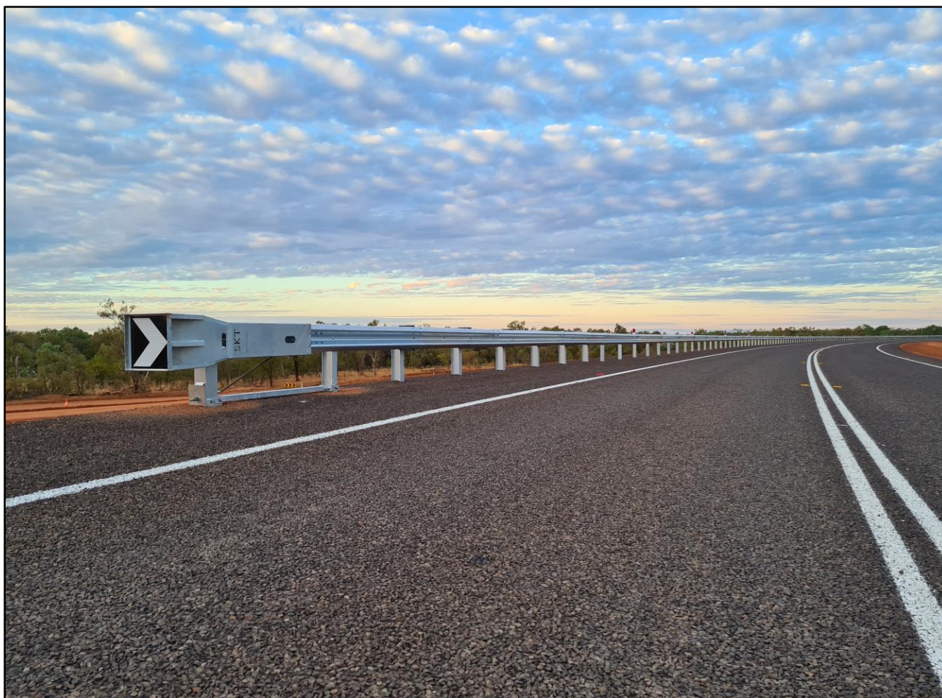
Figure 5: RamShield® W-Beam, Attachment to MSKT.
