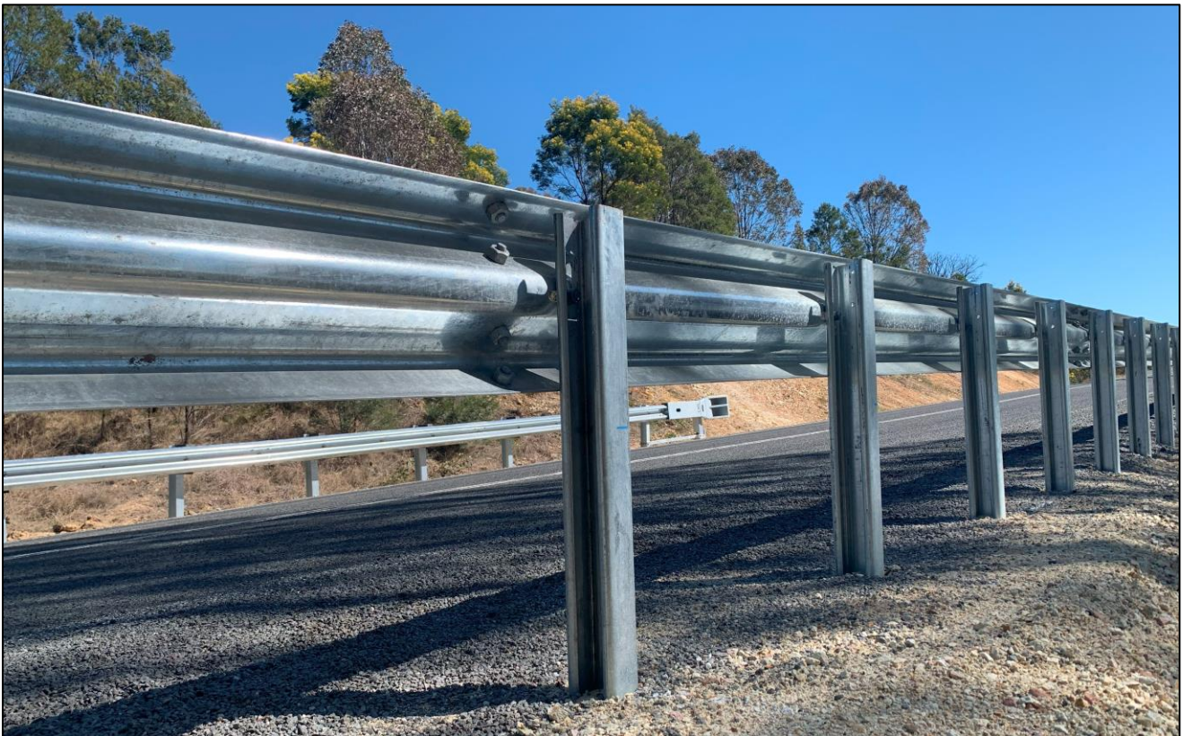
Figure 4: RamShield® W-Beam, Reduced Post Spacing
