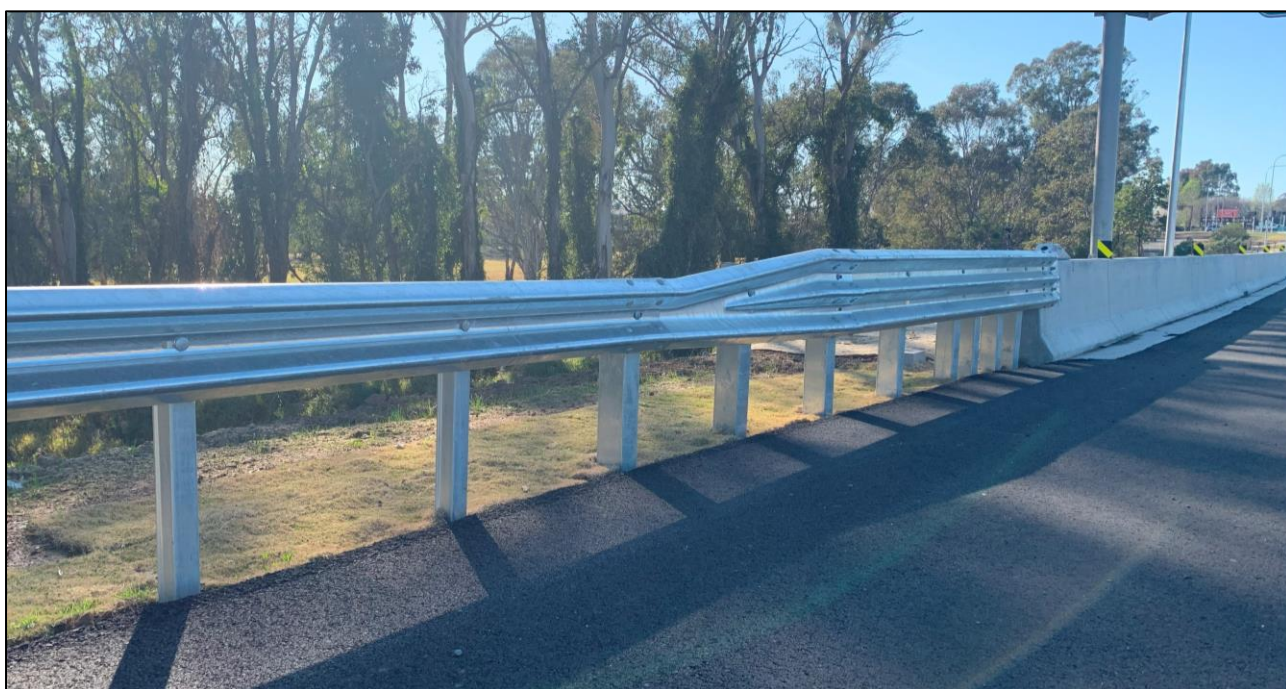
Figure 6: RamShield® Transition, Connection to RamShield® W-Beam
