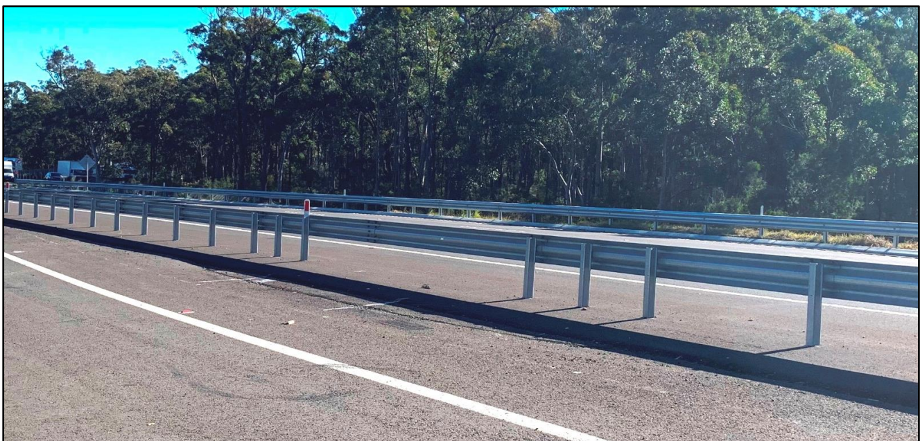
Figure 3: RamShield® W-Beam, 6m Span without Posts.
