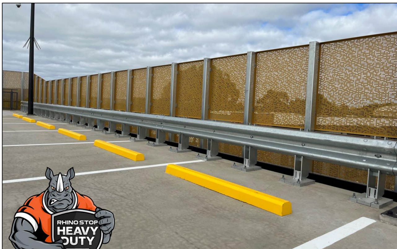
Type 2 Guardrail with offside handrail 1100mm high
