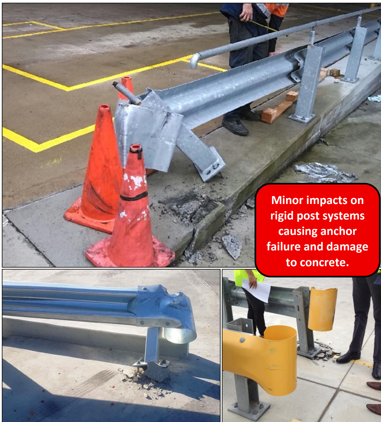
Figure 2: Impact behaviour of rigid post systems.
