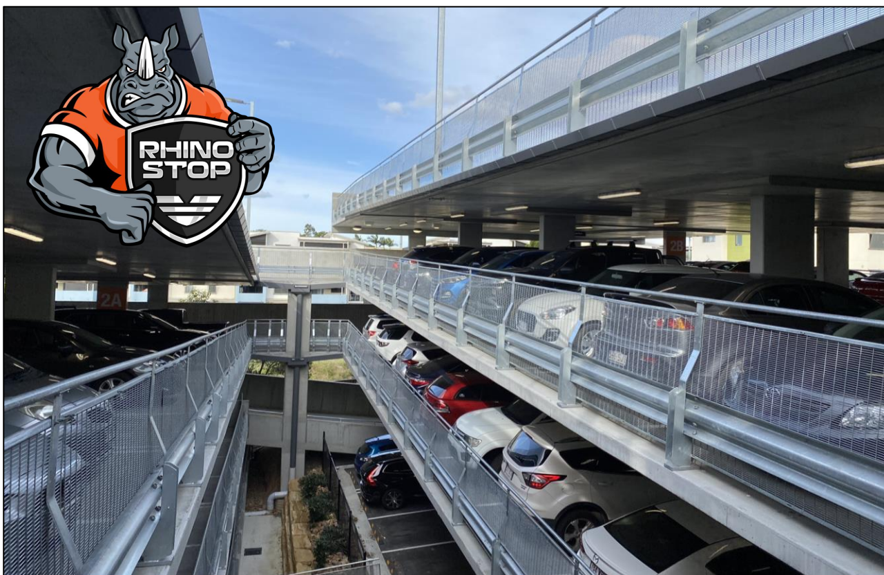
Type 2 Guardrail with offside handrail 1100mm high
