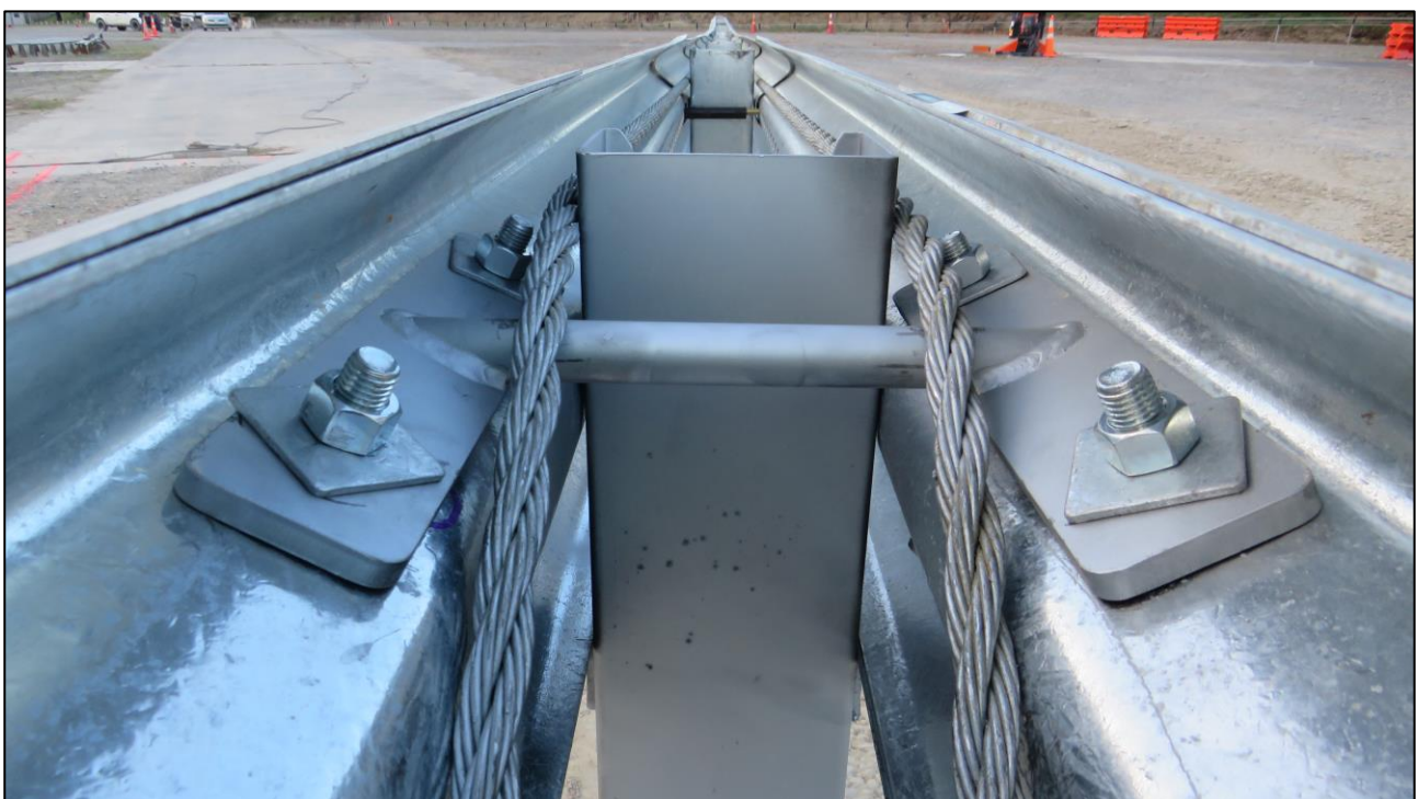
Figure 13: Cable Assemblies Passing over Cable Assembly Brace
