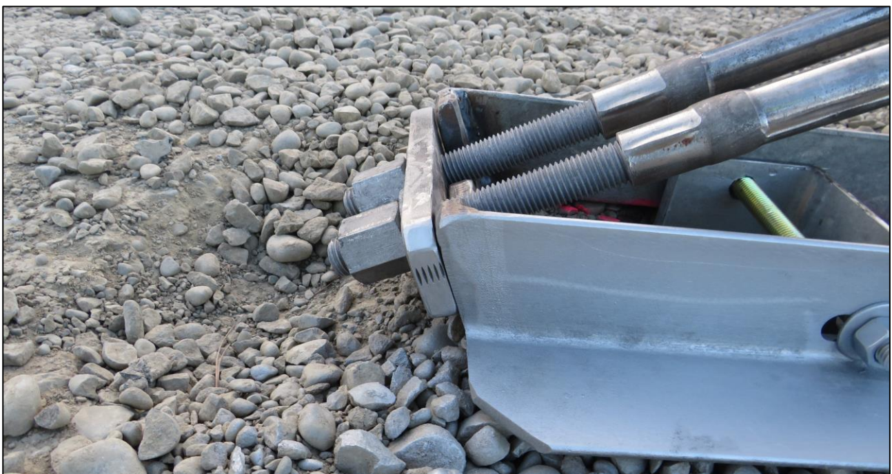
Figure 14: Securing Cable Assembly at Nose of Terminal with the Cable End Plate
