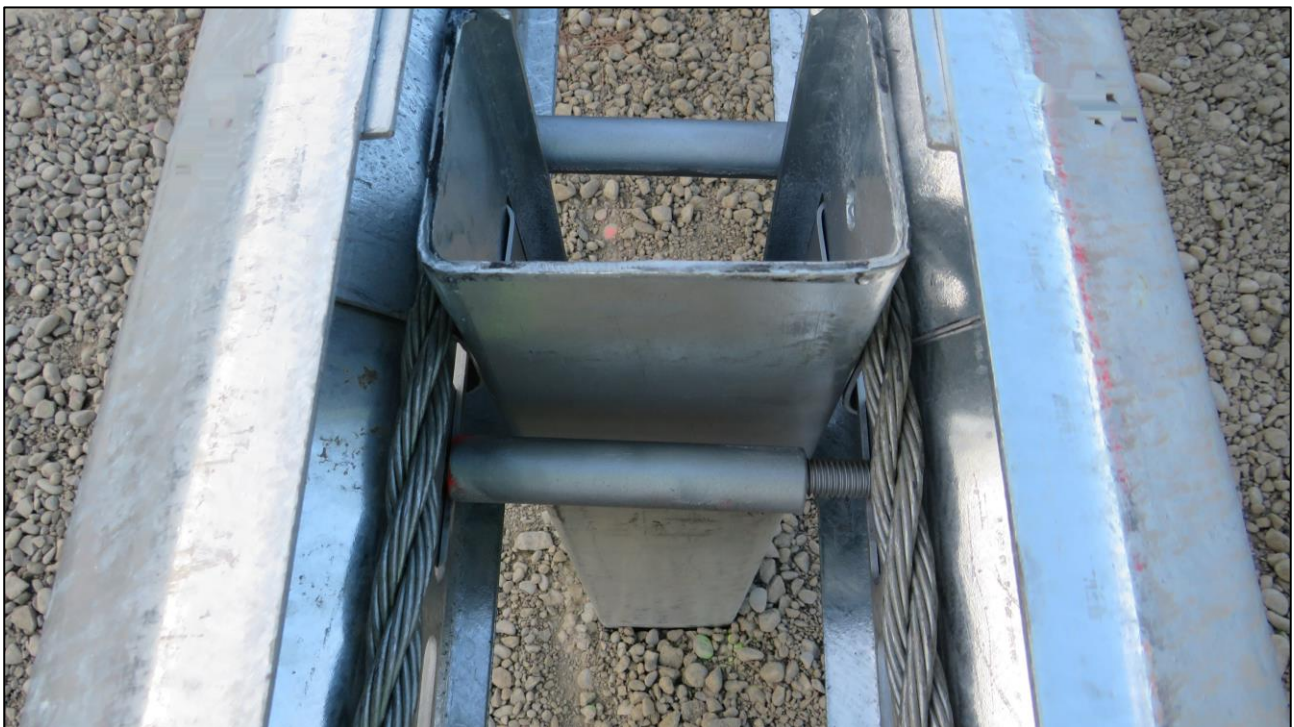
Figure 12: Positioning of Cable Assemblies between C-Posts and Rail Assemblies
