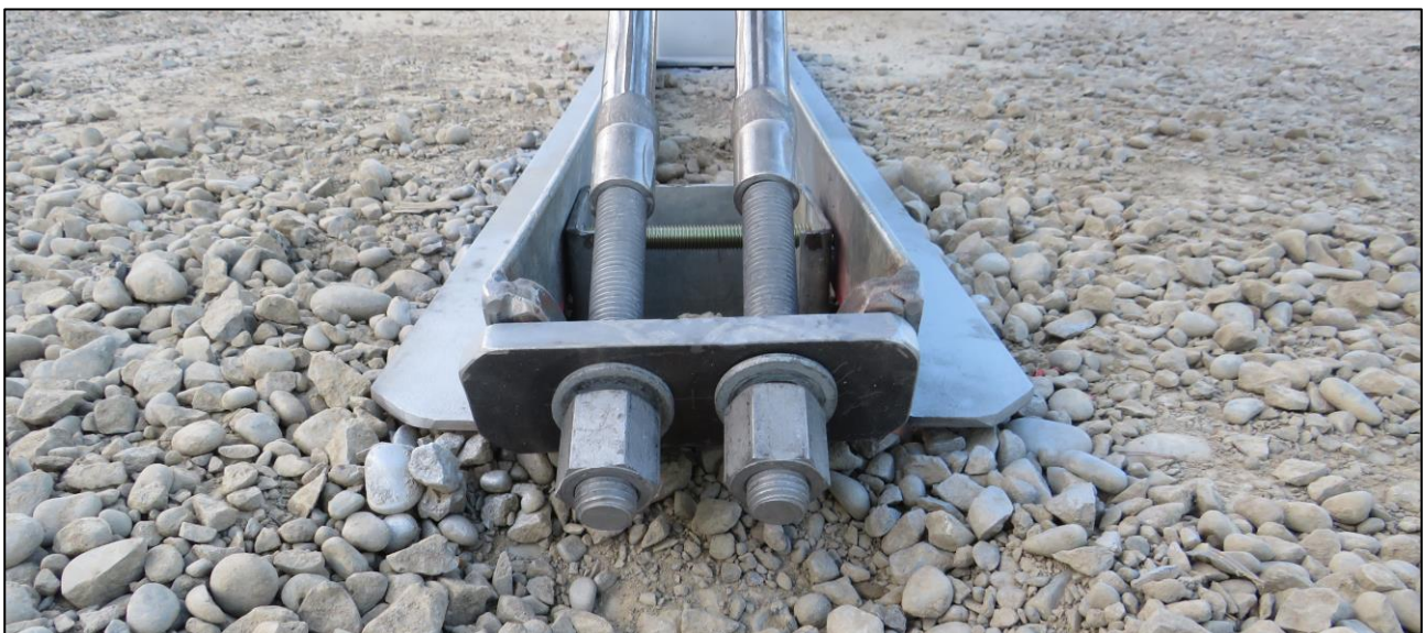
Figure 15: Assembled View of Cable Assemblies at nose of terminal
